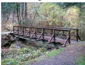
A new bridge now crosses Jackson Creek on the Sarah Zigler Trail. After over 15 years of use, the original foot bridge was determined to be suffering from long term exposure to the weather, dry rot and age. The bridge replacement, which took place last fall, was a joint project between the City of Jacksonville and The Jacksonville Woodlands Association.
