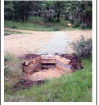
This wooden cut-off collar will help collect running water, and force it through the French drain (gravel-filled ditch) on its journey down the drainage..
